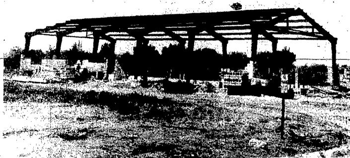
WORKMEN WERE BUSY this week on a new steel span building that will be the new home of Morris Machine shop. The steel and concrete structure is being erected between South Main and South Pearl. Owner Stanley Morris said he expects to occupy the new building about Aug. 1. The fire-proof, 40x100-foot structure will have an insulated steel roof with 10 skylights, two 16-foot drive-in doors and four walk-in doors.
